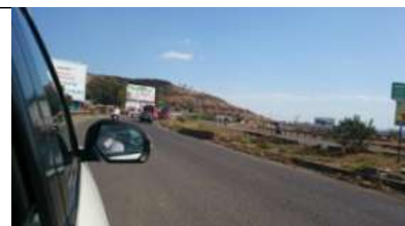
Incomplete part of the 6 laning
